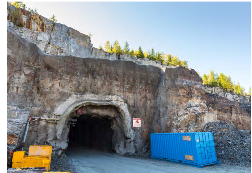
Example of ramp portal
