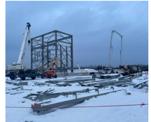
Shaft and Hoist Structures
