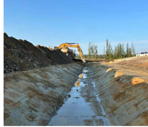
Site roads, pads and ditches
