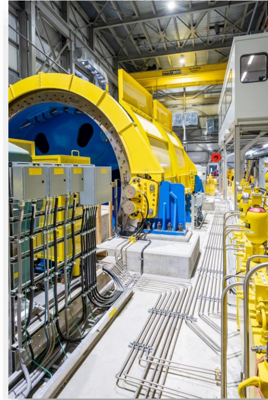
INSIDE HOIST ROOM
