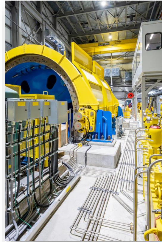
INSIDE HOIST ROOM
