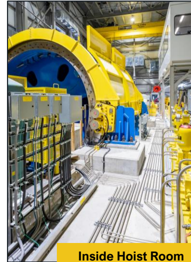
Inside Hoist Room
