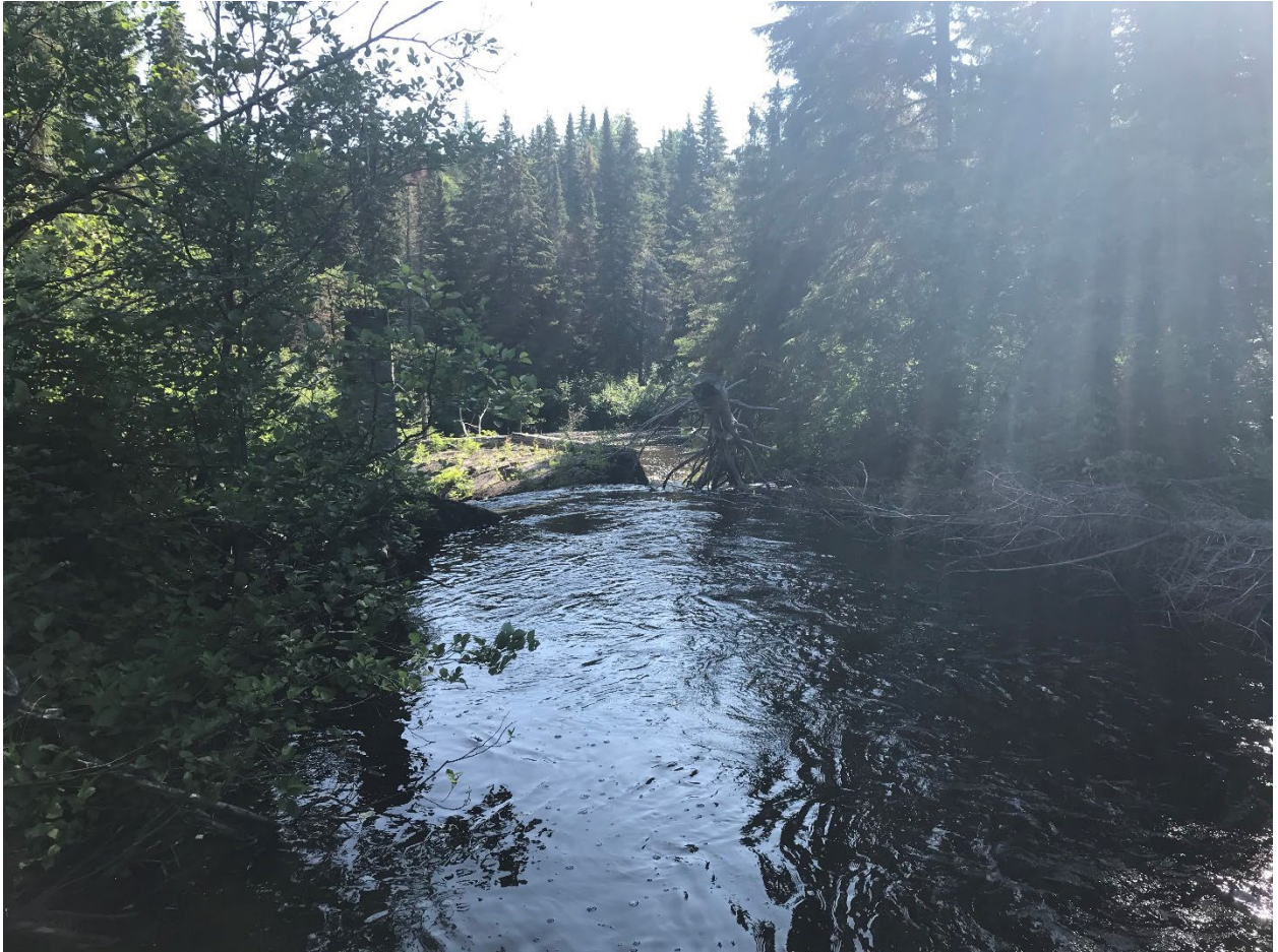
Figure 14: Victoria Creek Dam, July 2019
